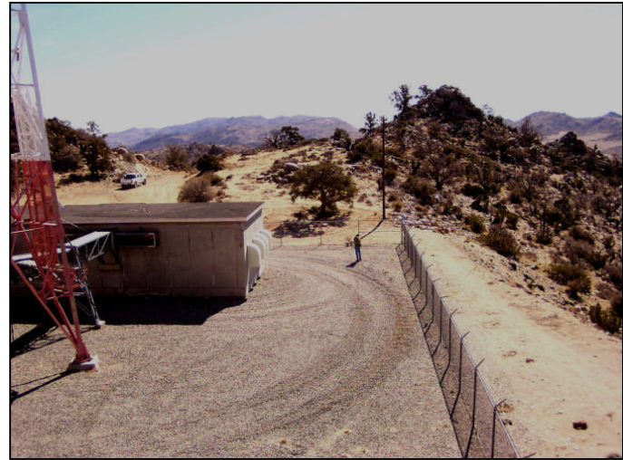
Photograph 4: View toward Joshua Tree candidate location, facing southwest.
